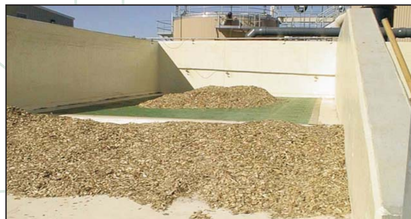
Bio Floor™ system installed in 3 sided concrete vault loaded and unloaded from open side.
