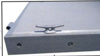
Mooring Cleats Bolted Through Dock Frame
